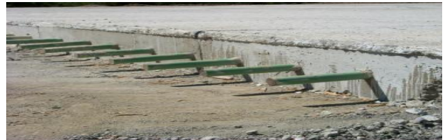
Steel Load Transfer Bars
